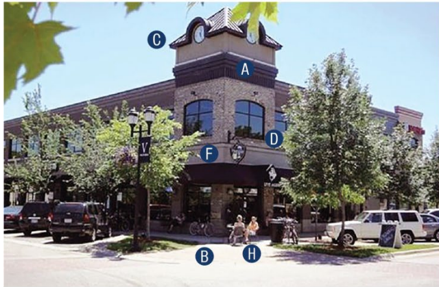
Figure <>: Primary Building Entrances
