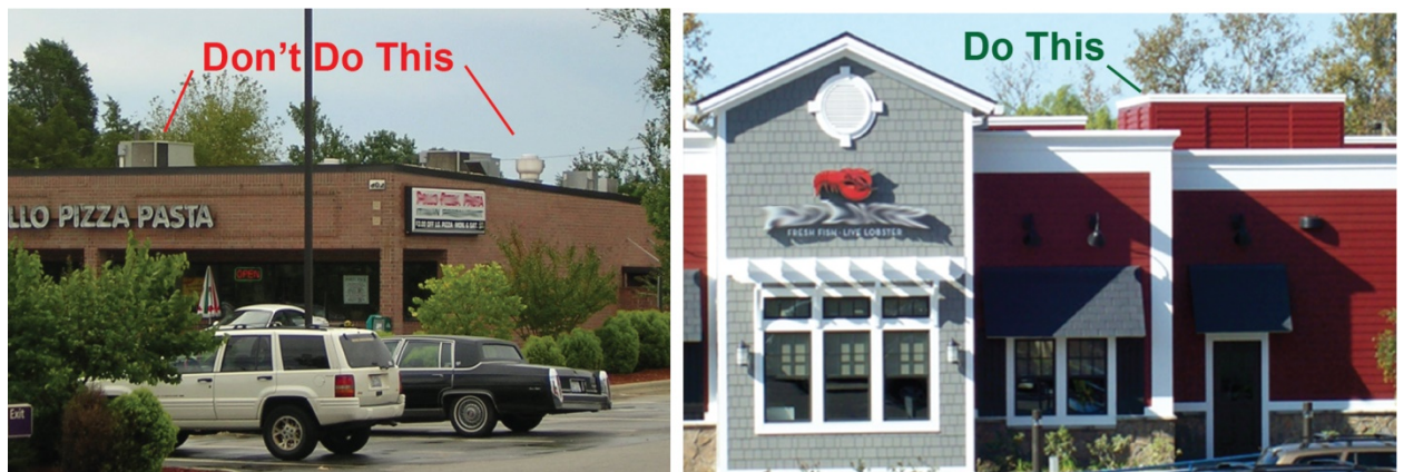
Figure <: Rooftop Screening
